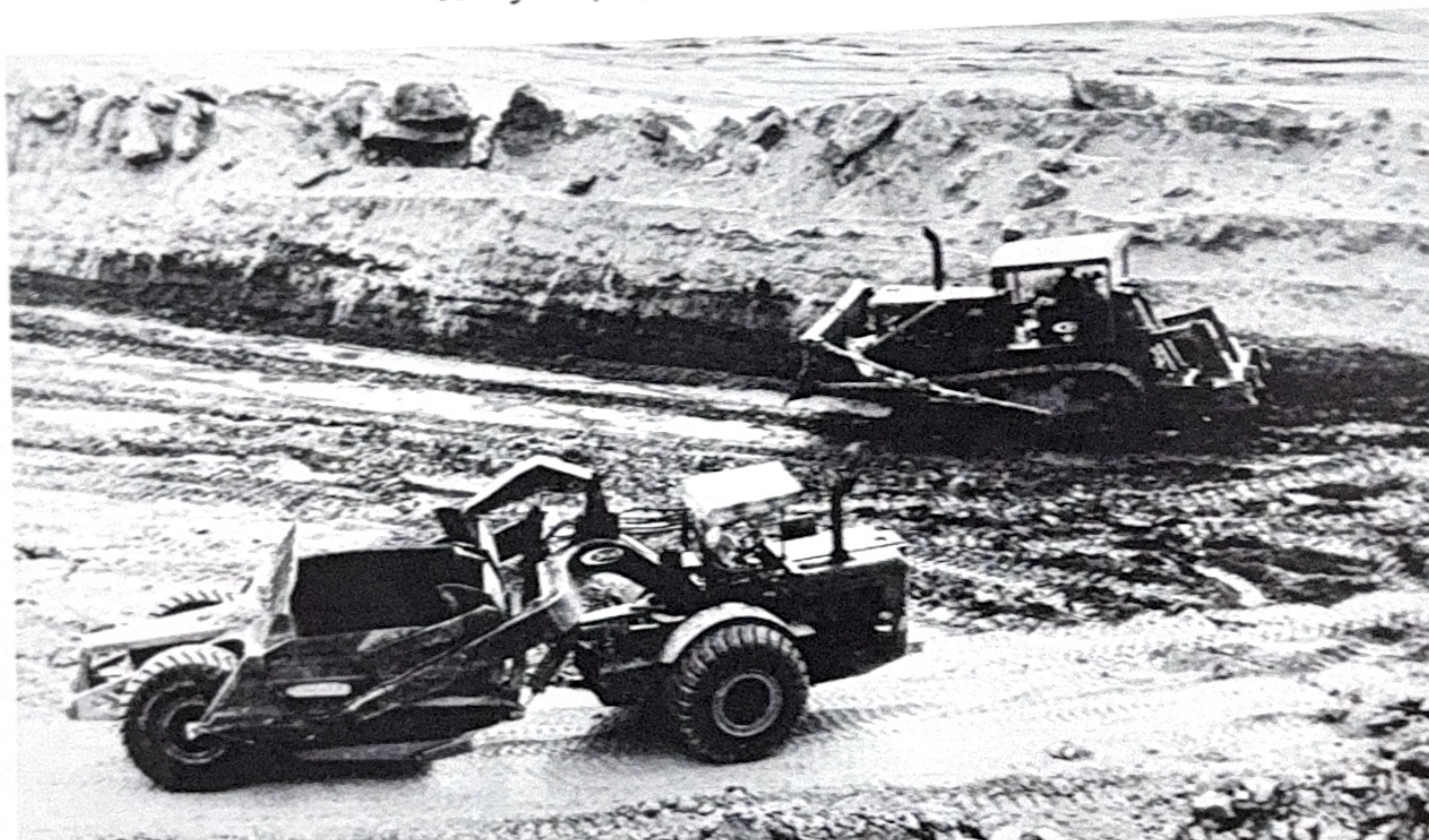
To speed loading of material, a 22-ton crawler ripped the rocky cut area prior to action by the scraper ready in the foreground.
