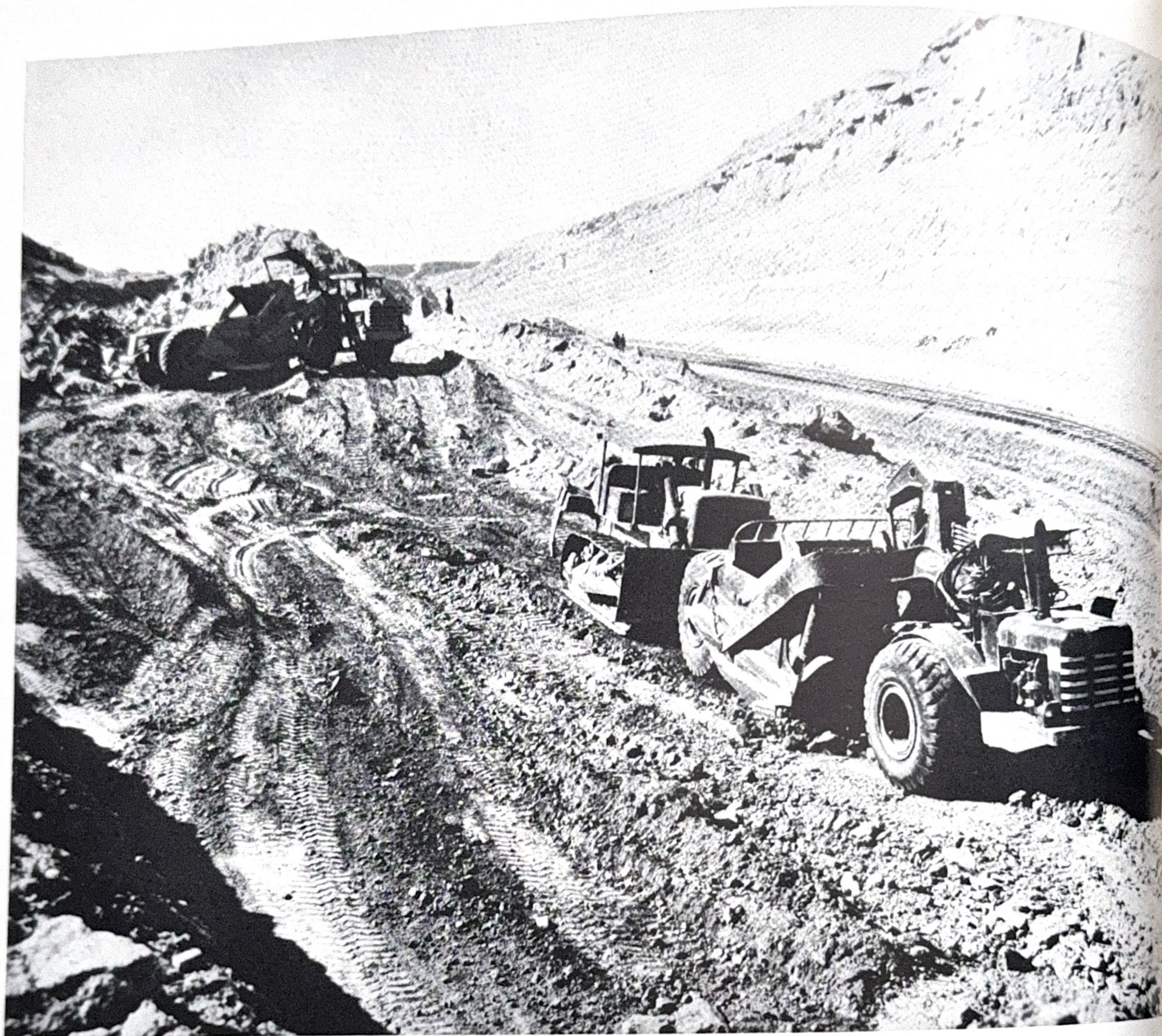
A crawler push-loaded a scraper while another scraper awaited its turn on the port project site in Angola.
