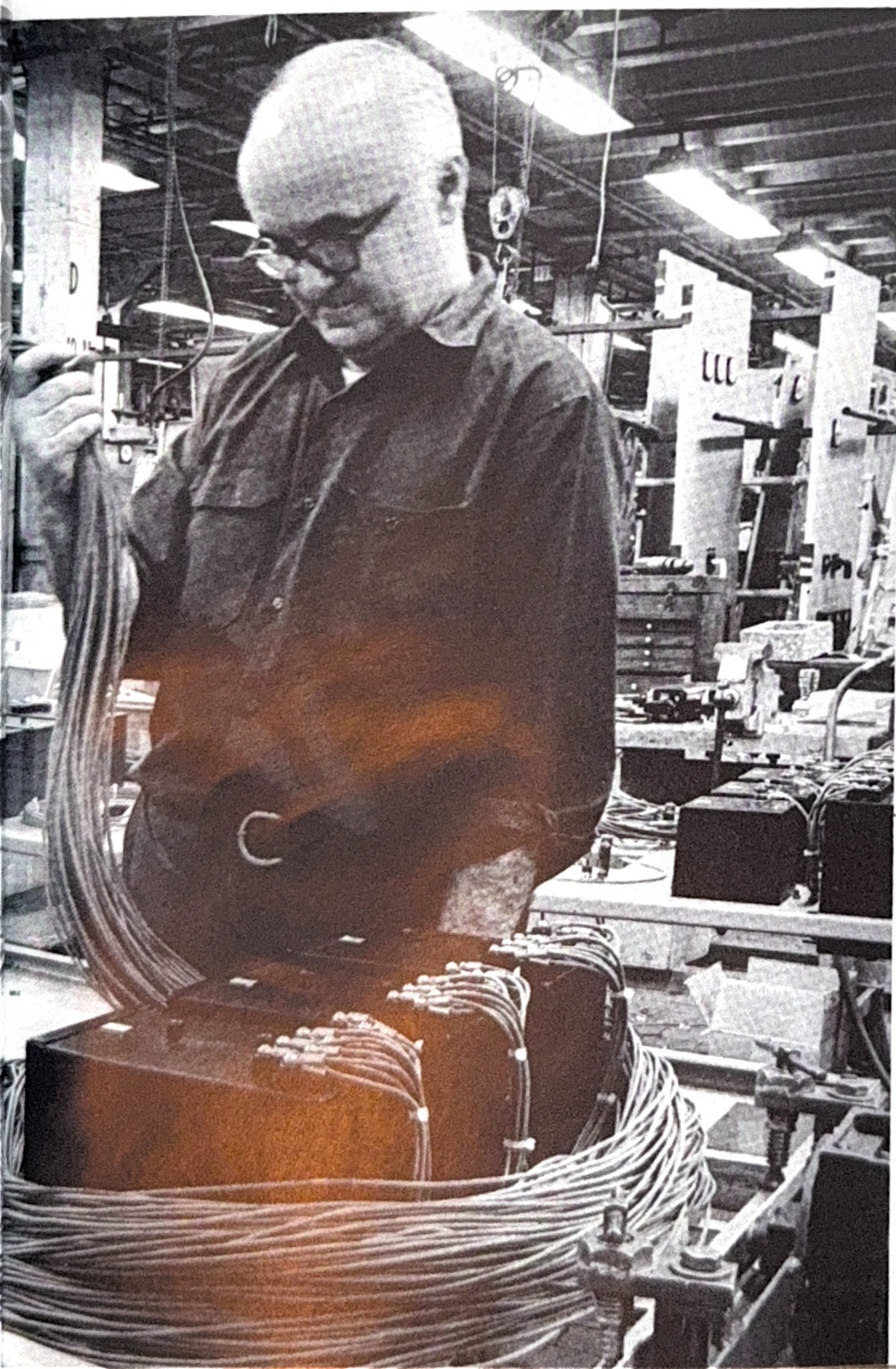
Hundreds of feet of wire are used to connect the functioning, metering and control components. This bundle handled by Ratko Pavlovich (foreground) and Earl McGivern contains 80 strands.
