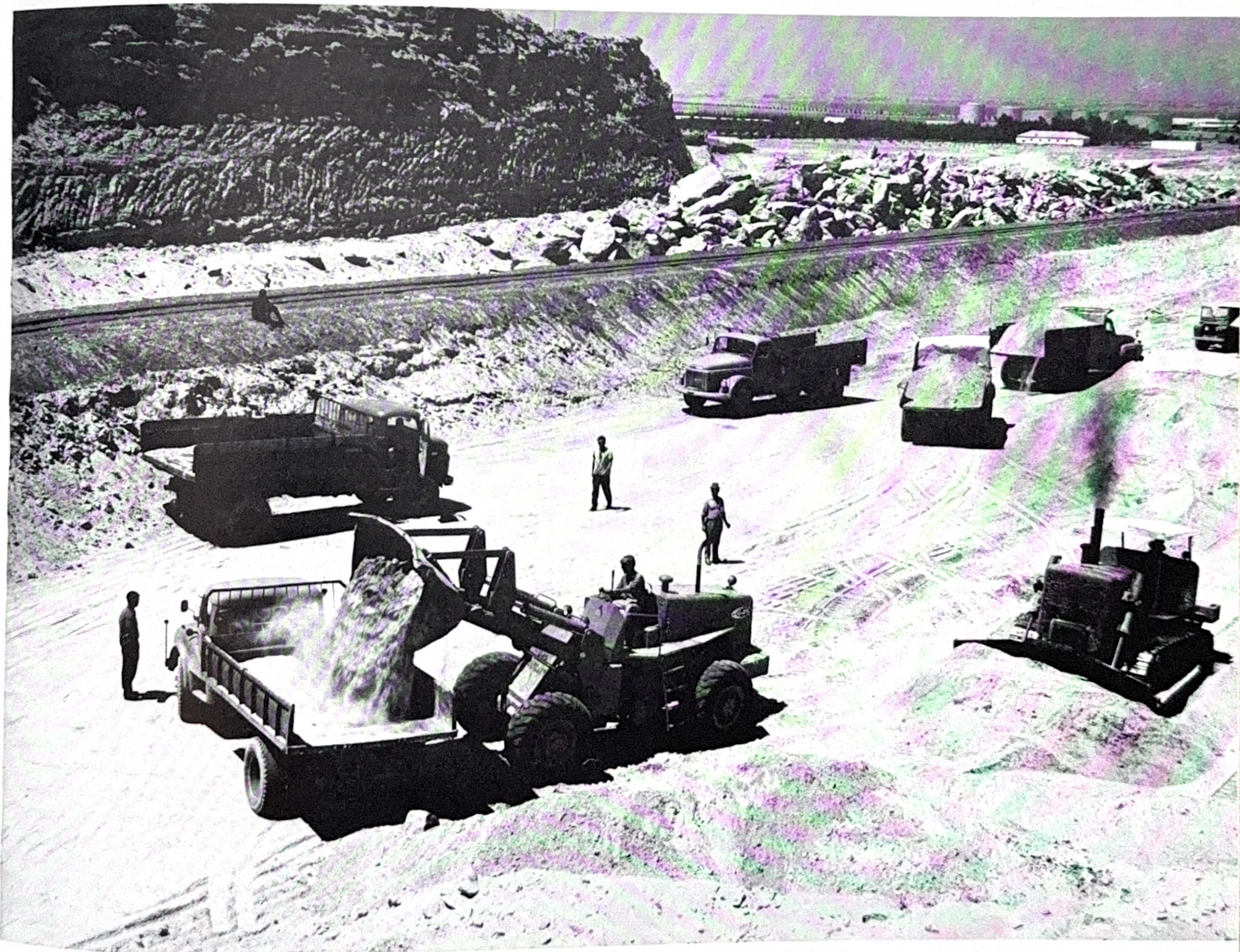
Rock and sand spoil, pushed into piles by a crawler, was dumped into a truck by a wheel loader.
