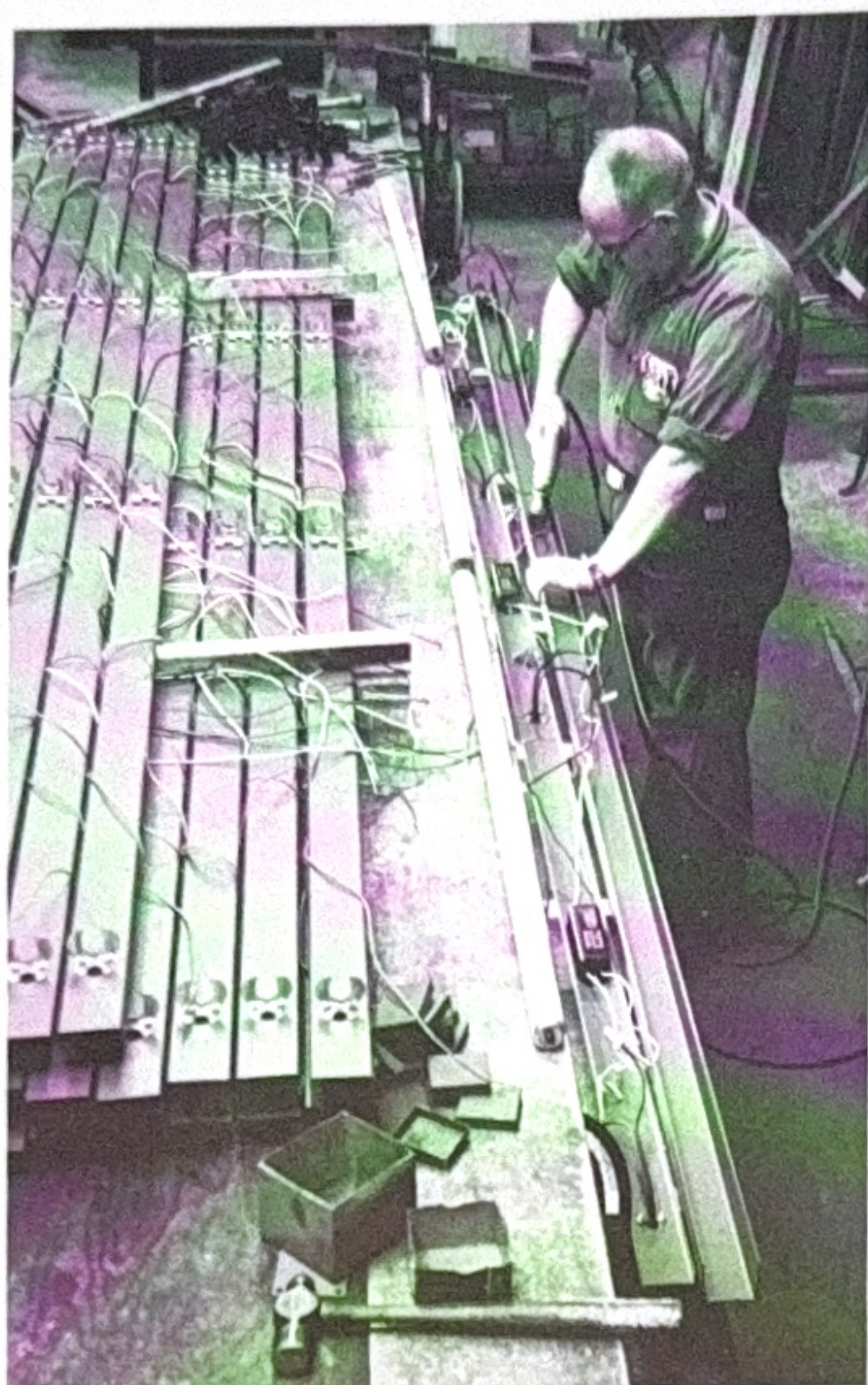
Hundreds of intricate steps are necessary in the construction of each Ferris wheel. At left, Gerald Brockhaus wires for bulb and neon electric lighting; at right, Fred Stewart finishes decoration of a seat.
