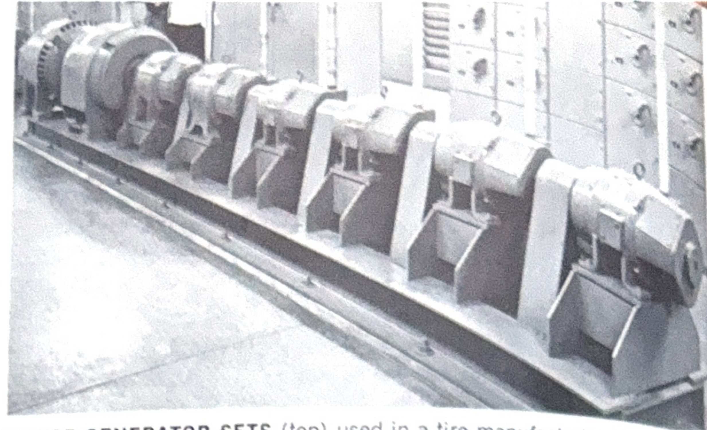
MOTOR-GENERATOR SETS (top) used in a tire manufacturing plant in Ohio. Lower photo, this axial compressor furnishes air at a Southwest oil refinery.
