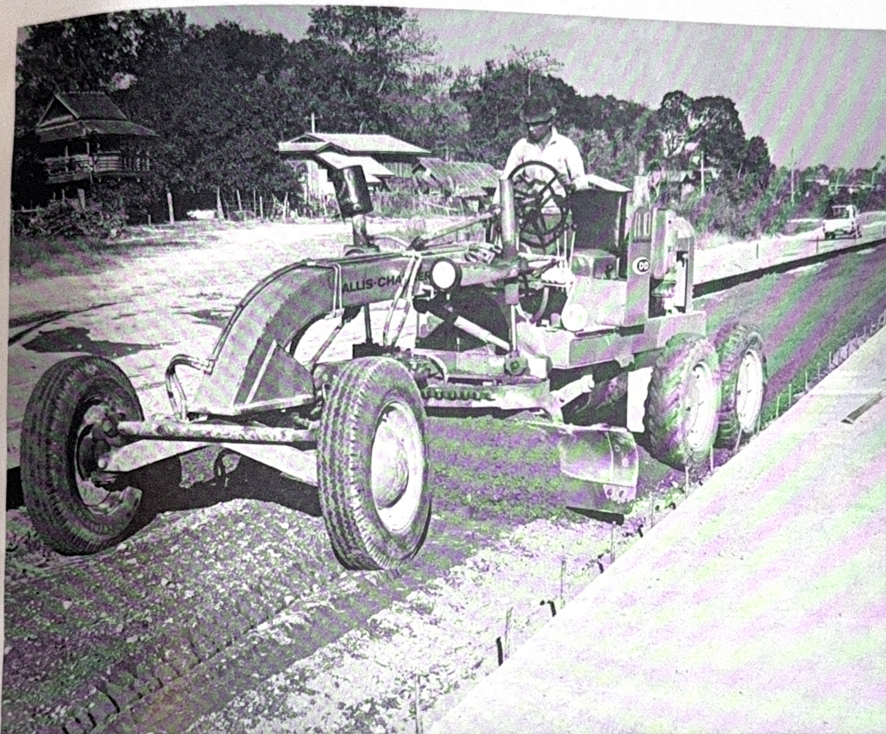
A grader spreads base material. When necessary, construction in this location means improvising, such as front tire replacement by a truck wheel—complete with the hubcap.
