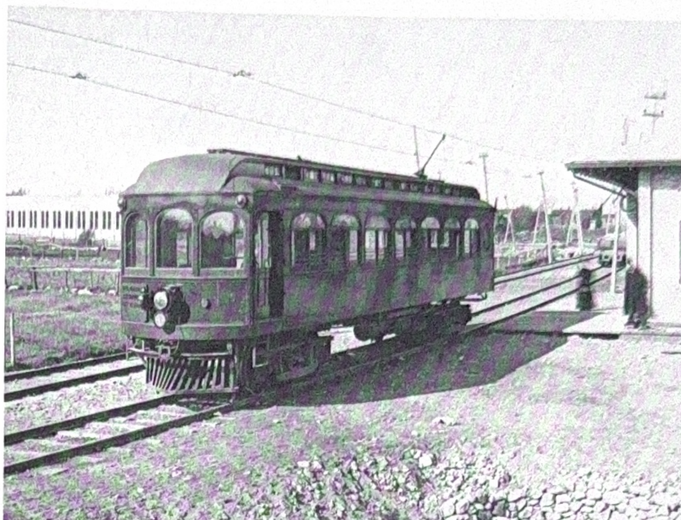
This 1907 vintage interurban railway car and thousands of others like it were equipped with Allis-Chalmers built air-brakes. Compressors for the brakes, such as the one pictured above, were mounted beneath the cars. Boarding and exiting passengers had to step up and down nearly three feet.
