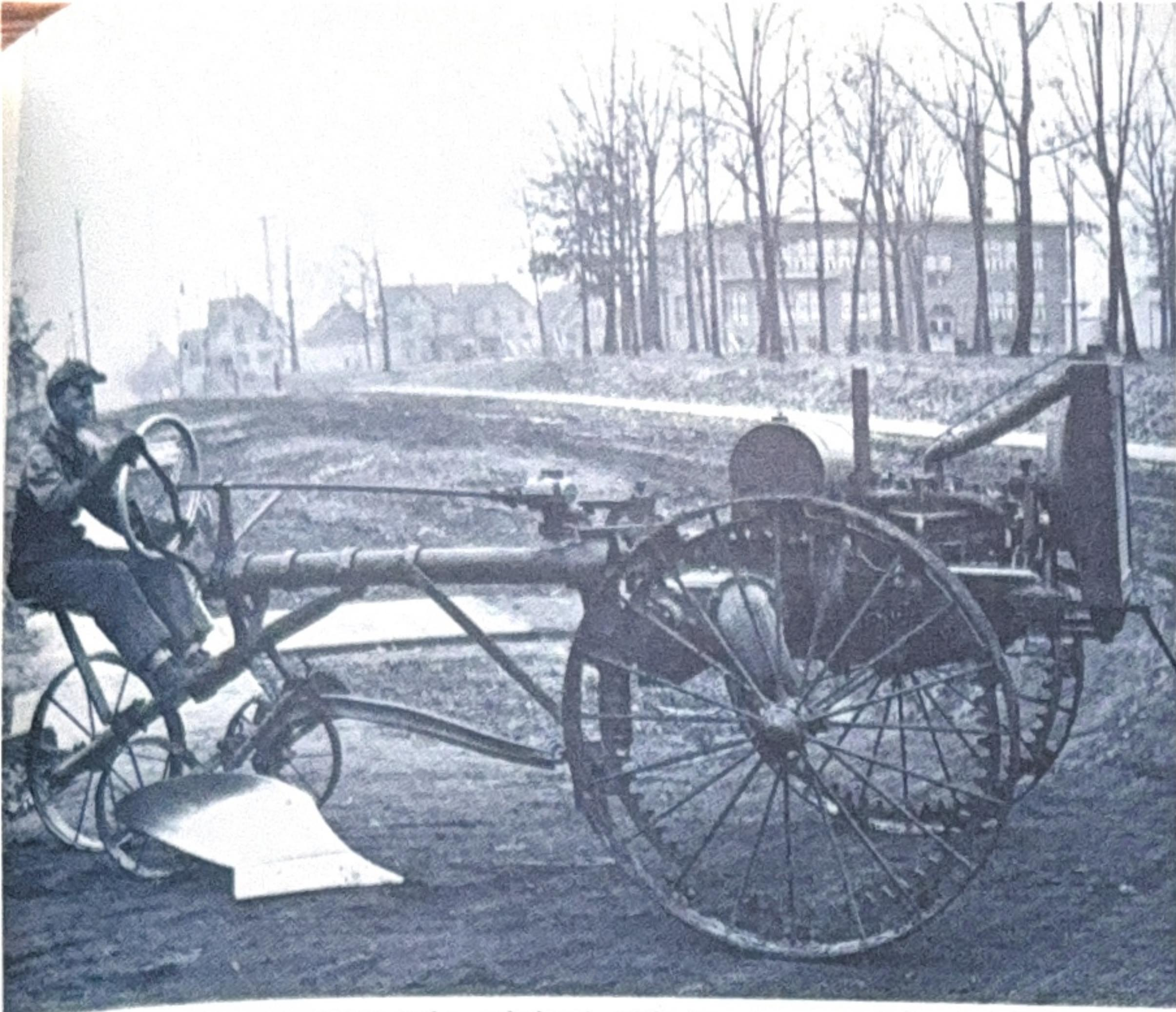
**IF YOU CAN REMEMBER** this original Allis-Chalmers all purpose tractor, you're due for a 50-year pin soon. The unit was one of our Company's first tractors, in operation during the World War I year of 1915. This model was equipped with a one-bottom 16-inch plow. It had a top horsepower of 12, and worked at a speed of about 2 miles per hour. Compare it to today's sleek and powerful "One-ninety" below — 90 hp, and operational speed of up to 15 miles per hour.
