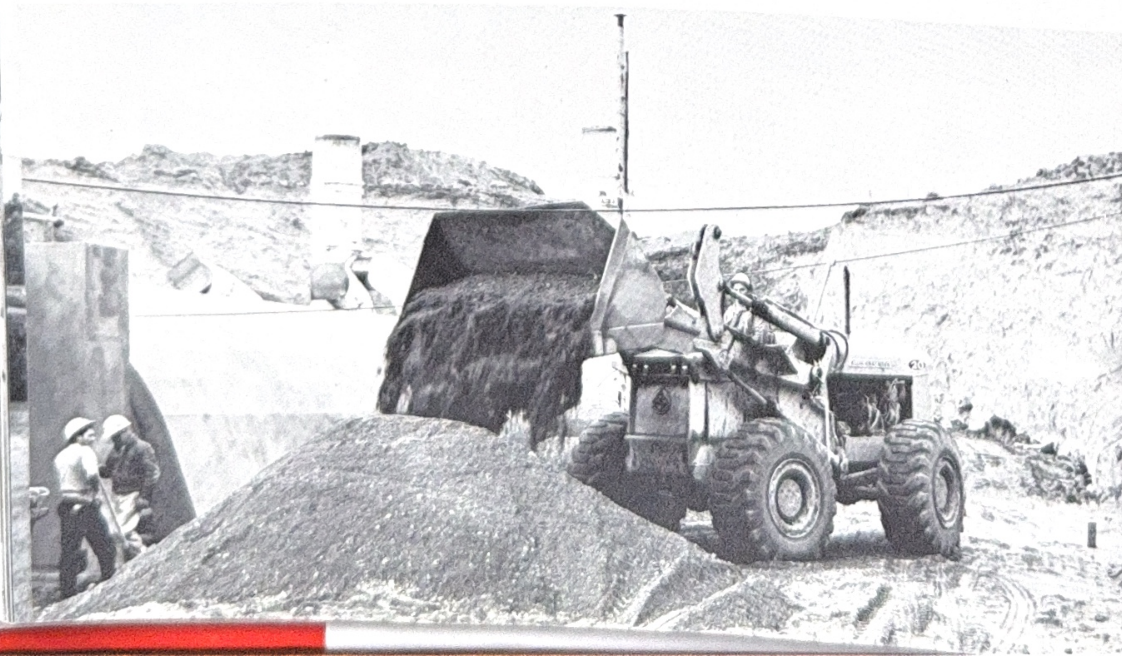
An A-C tractor loader back-fills at a completed Minuteman launch control center capsule near Minot, North Dakota.
