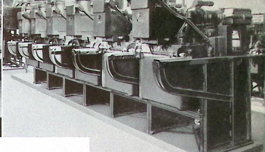
Six Armoclad Switchgear units feeding a continuous hot strip steel mill.
