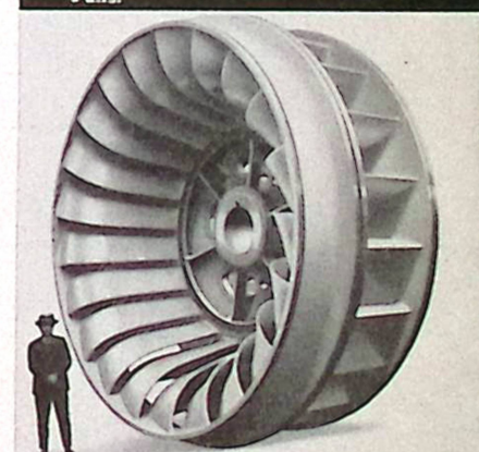
This cast steel runner from one of the Niagara Falls turbines weighs 100,000 pounds.
