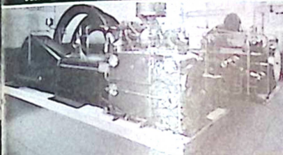
Two Allis-Chalmers 500 KW Cross Compounded Engine Generator sets.
