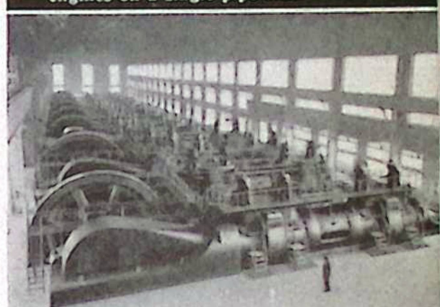
An A-C Triplex oil engine and duplex double acting plunger pump. The Company has installed 180 of these engines on a single pipe line.
