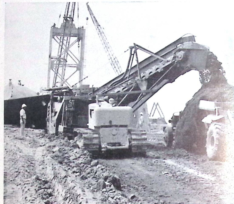
An A-C crawler tractor is used, above, to push loader which fills motor wagons in ground-clearing operation at refinery. Big ditch, below, carries part of the 48 miles of concrete ducts encasing 200 miles of electrical lines on the site. The refinery will use as much power as a city the size of Gadsden, Ala. (55,000 people).
