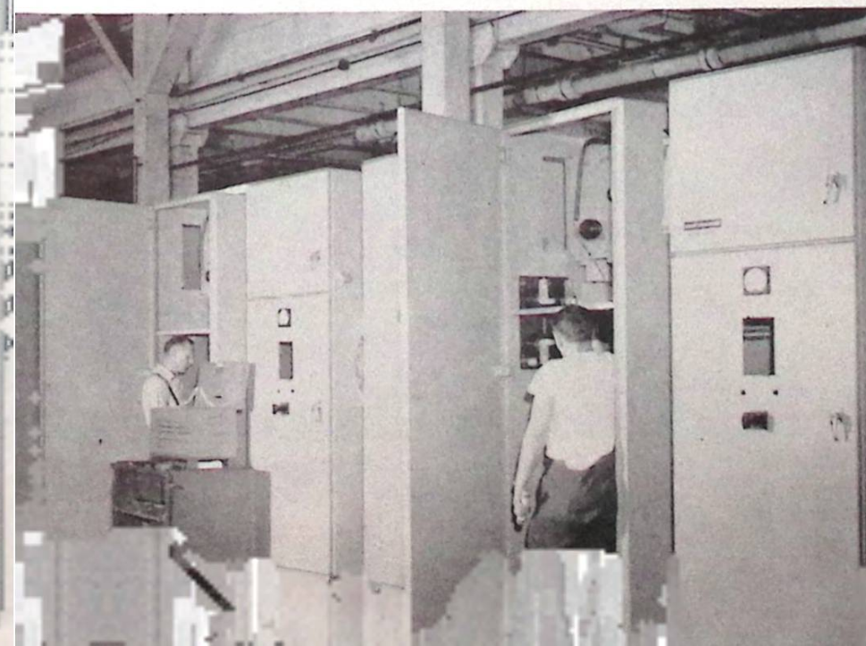
Portion of the A-C metal-clad switchgear installed in the refinery's power station is shown above with Hal Lanphear (left), Philadelphia district office representative, and a Delaware Power & Light Company engineer looking it over. Below, Adolph Zabana (left) and Emil Ruck are working on the "assembly line" production set-up used at Hawley to produce more than 100 Type HALC motor starters for the water refinery.
