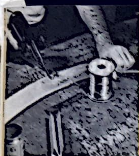
Joe Prohaska solders a static ring at Terre Haute.
