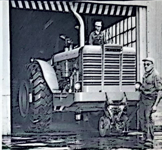
At Cedar Rapids Works, George Sheets (right), tractor assembly man, and William Peterson, tractor assembly inspector, roll a TS-360 off the assembly line. After the scraper bucket is attached, the unit will be ready for shipment to an Allis-Chalmers customer.
