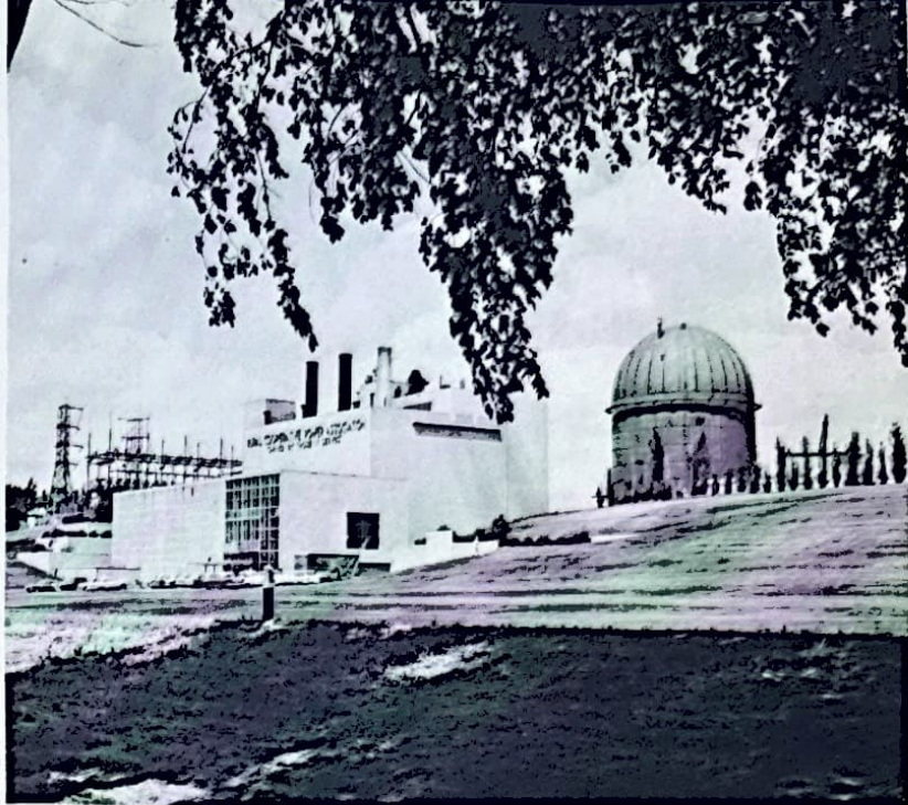
Scheduled to go into operation soon is this 22,000-kw reactor built by A-C for the Rural Co-operative Power association, Elk River, Minn. The unit operates with existing plant facilities and will produce steam at same temperatures and pressures as that from the existing boilers.
