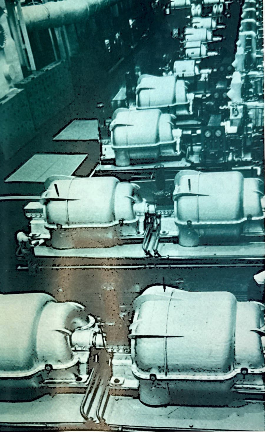
These Allis-Chalmers compressors and steam turbine driven exhausters are installed at the Willgoos Turbine Engine Test facility powerhouse in East Hartford, Conn. The laboratory, owned by Pratt & Whitney Aircraft division, United Aircraft Corp., is capable of testing turbojet, turboprop and ramjet engines at simulated altitudes up to 80,000 feet and at speeds in excess of Mach 3, or three times the speed of sound.
