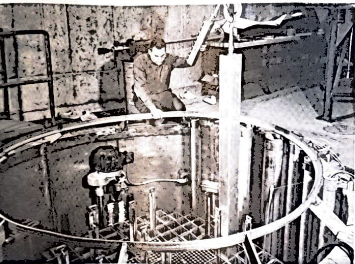
Overhead crane is used to lower nuclear fuel element into core of critical test facility at Greendale nuclear research facility.
