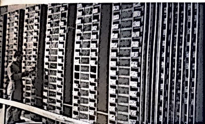
Fuel storage vault in the critical facility building at Greendale houses nuclear fuel elements used to make up the "working" portion of larger fuel control rods.
