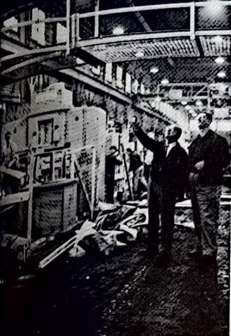
A section of the overhead conveyor and guard must come down to permit this machine to be moved to a permanent location. George Plopper, Tractor shops safety supervisor (pointing), asks Frank Janda, millwright foreman, what the job entails. Steve Stano, millwright, uncrates the new machine on the flatcar in the background.
