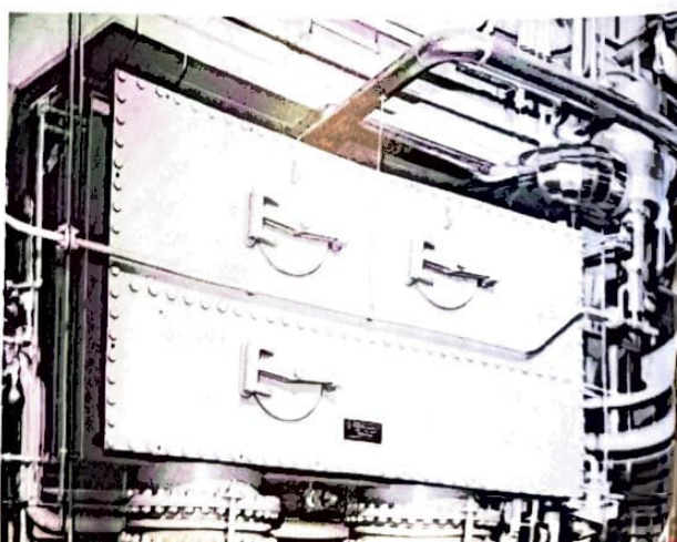
A 19,000 square foot Allis-Chalmers condenser is at work at the new Rapid City plant of the Black Hills Power and Light Co. The firm serves six western South Dakota and three eastern Wyoming counties.
