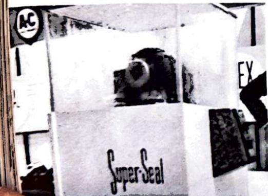
This Super-Seal motor provided an effective demonstration of its insulation. The motor was enclosed in a glass case and subjected to sprays of water while it was running.
