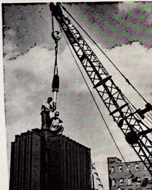
Martha J. Duffin, Pittsburgh — Placing bushing on top of power transformer. 4 x 5 Speed Graphic, F 22, 1/100 sec., Tri-X film, one No. 25 photoflash lamp for fill-in.
