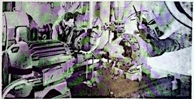
A-C pumps, found in abundance in the paper mill operation, are adapted to the many different needs of the industry. Here unscreened bleached stock is being pumped to the flat screens.
