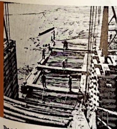
The pulpwood logs begin their long ride through the paper mill here at the jackladder. They have been floated downstream to the mill and are now ready to be debarked.
