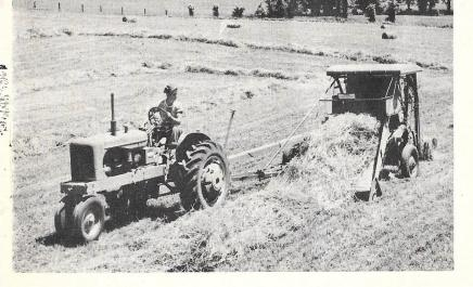
Double windrows cut in half the amount of field travel both in baling and collecting bales later.
